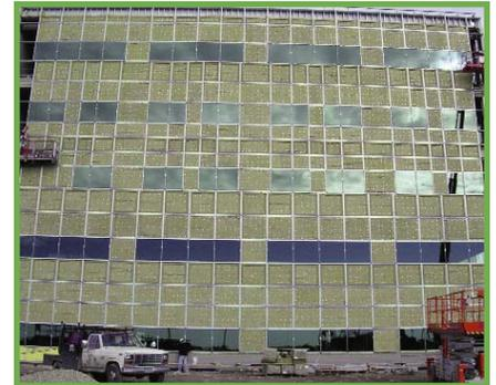
This facade shows insulation pin welded to back pans prior to being covered with metal wall panels. Alberta Children's Hospital, Calgary, Alberta. Kasian Architecture.
