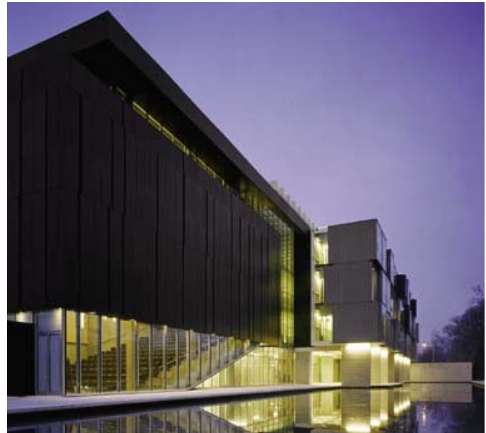
Black anodized Alumaspan™ wall panels on facade over reflecting pool. Perimeter Institute for Theological Studies. Waterloo, Ontario. Saucier & Perrotte Architects.
