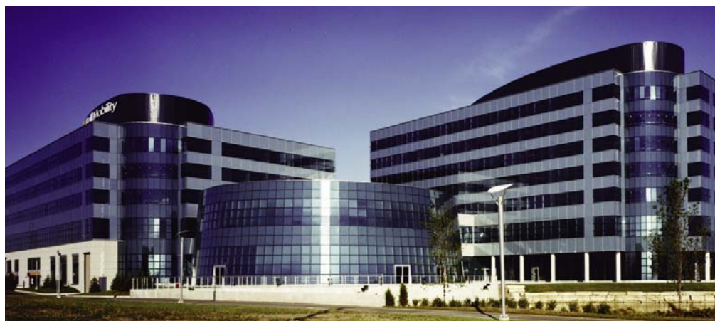
Alumaspan™ Preformed Aluminum Wall Panels, used in cylindrical building. Bell Mobility Headquarters, Toronto, Ontario. Page + Steel Inc.
